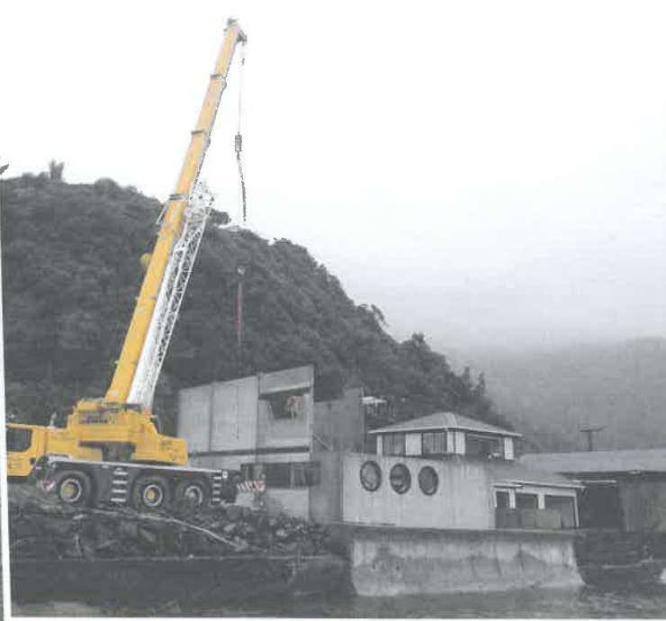
The crane sits on sanctuary land while it drops a concrete wall for Phil's house into place. Photo: Bruce Sedcole
