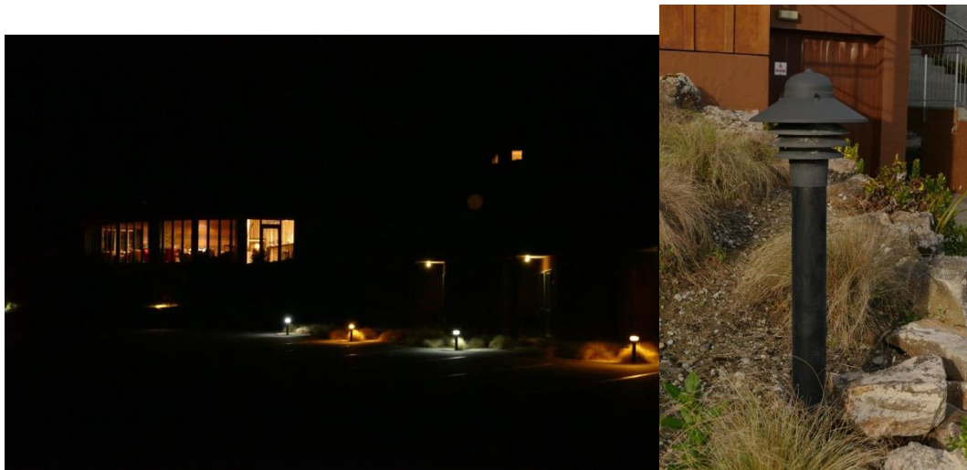
Figure 7. Left, the Punakaiki Resort at night showing the low light levels facing seawards. The room on the left is the main communal area including restaurant. Right, one of the path lights hooded to prevent light spill skywards, four of these can be seen in the photo on the left. Photos by Kerry-Jayne Wilson
